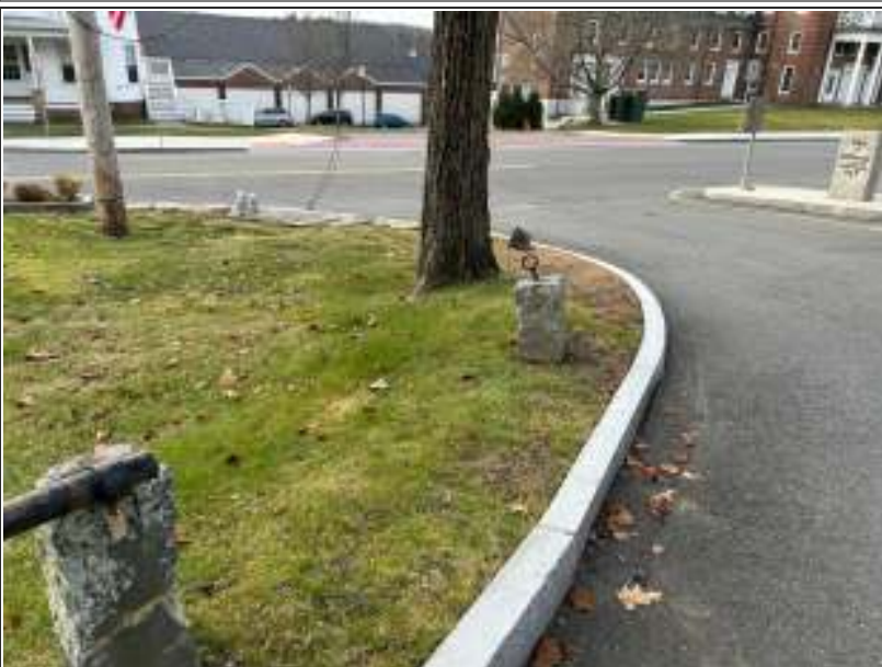
12/06/2023: View of Westerly End of Rail. Missing sections of rail and posts knocked over.(click on Photo to enlarge)
