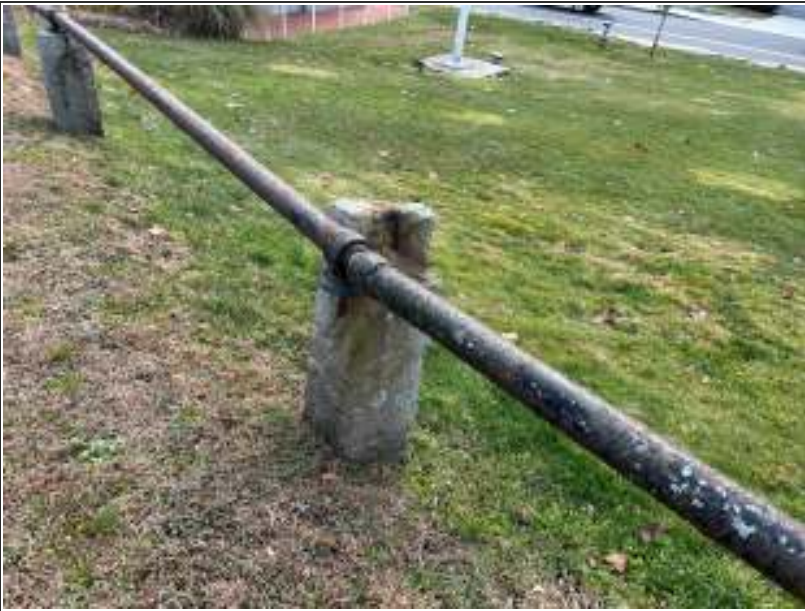
12/06/2023: Close up of failed Post-Rail Connection. (click on Photo to enlarge)
