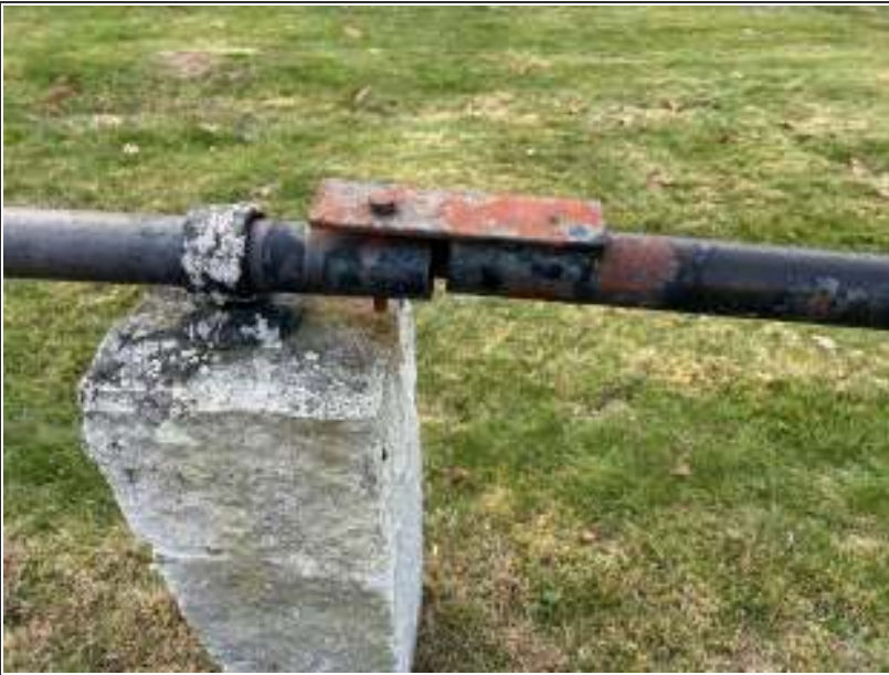
12/06/2023: Close up of misaligned rail "repair". (click on Photo to enlarge)
