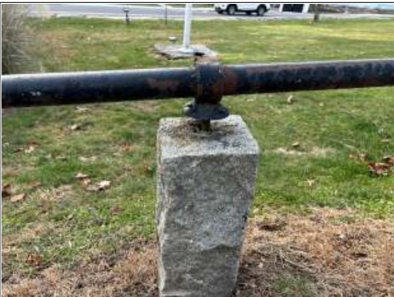
12/06/2023: Close-up of Rail - post failing (click on Photo to enlarge)
