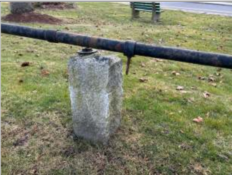
12/06/2023: Close Up view of Misaligned Post. (click on Photo to enlarge)
