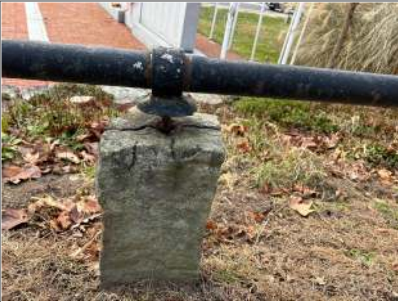
12/06/2023: Close-up of Failing Post-rail connection (click on Photo to enlarge)
