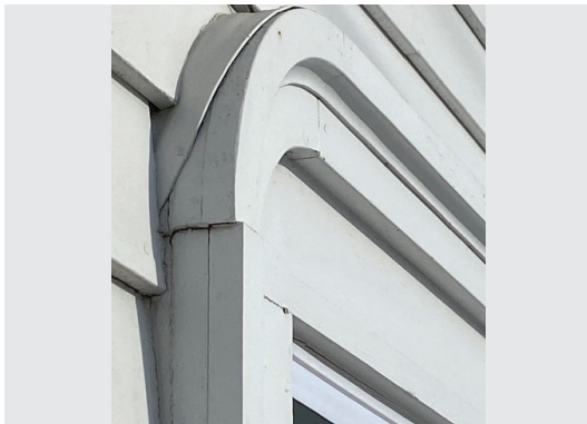
Image 24: Lead flashing over front door trim.
