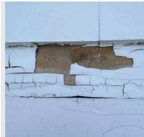
Image 18: Exterior Siding: Delaminating paint on clapboard. Alligating on clapboard below.
