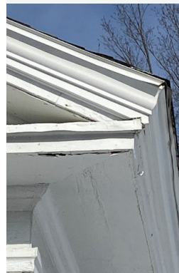
Image 21: Evidence of peeling paint at soffit.
