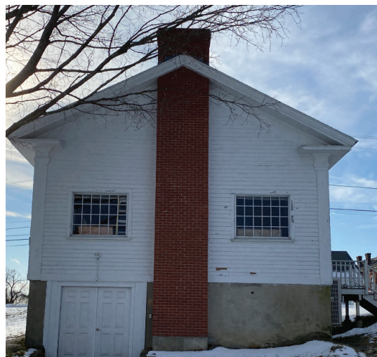
Image 7; North Elevation: Chimney penetrates the roof at the gable on the north side.
