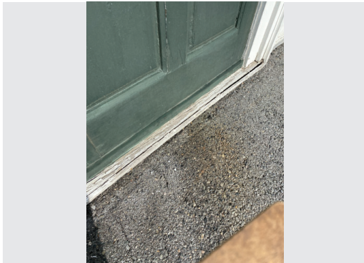
Image 23: Sill of Front Door--The sills at both front doors are deteriorating and should be replaced.
