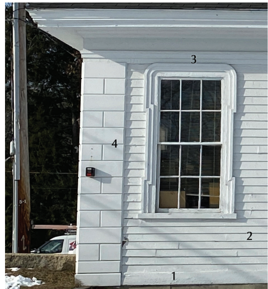
Image 12: East Elevation: Labeled exterior facade showing Greek Revival elements.
