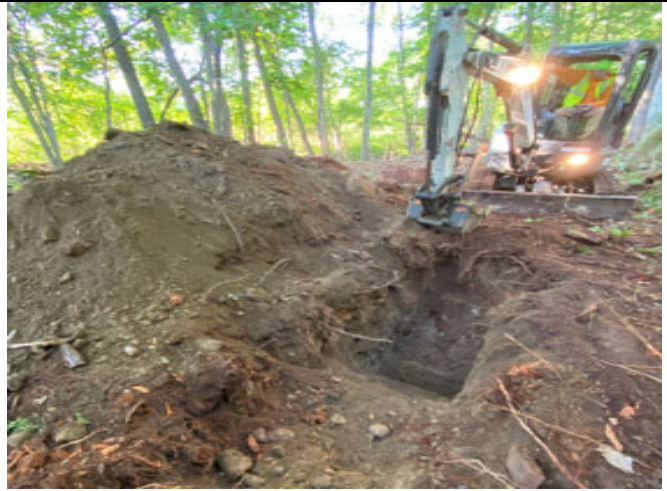
Photo 12: Test Pit TP(-20,100); refer to Figure 4 for location and Appendix E for a description of materials encountered
