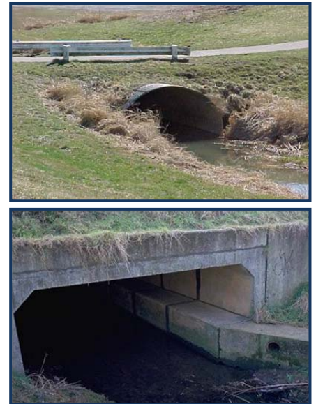
Before Mitigation and After Mitigation
