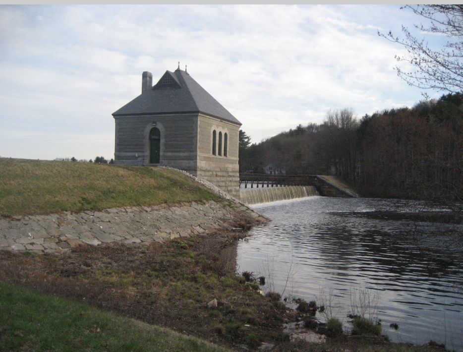
SUDBURY RESERVOIR DAM NO. 2
