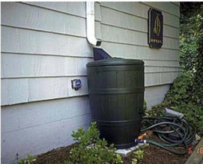
Figure 10: This rain barrel is used to collect rooftop runoff from a gutter/downspout system. Photo: EPA BMP Factsheets: On-Lot Treatment ( http://cfpub.epa.gov/npdes/stormwater/menuofbmps/post.cfm ).
