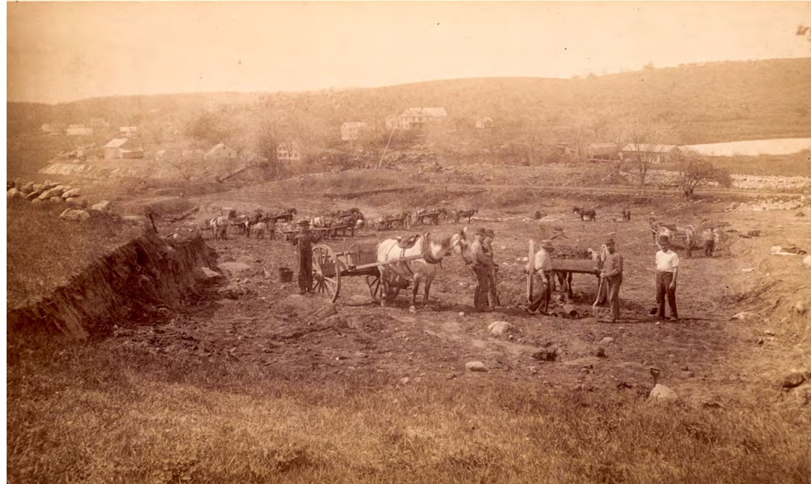
Sudbury Reservoir, construction, stripping north side hill, Southborough, Mass., ca. 1894
