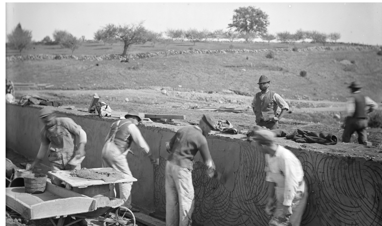
Sudbury Reservoir, plastering face of concrete core wall on north end of Sudbury Dam, from the west, Southborough, Mass., Sep. 26, 1896
